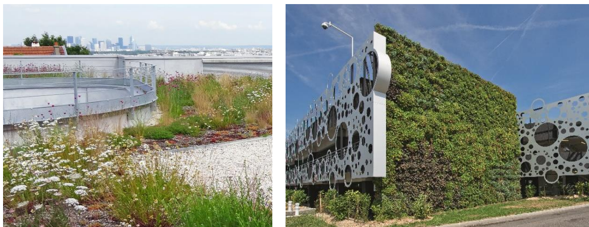
FIGURE 4 EXAMPLES OF CRITICAL INFRASTRUCTURES AND NBS: THE FIGURE ON THE LEFT SHOWS THE PERCY MILITARY HOSPITAL IN CLAMART (FRANCE), WHILE THE FIGURE ON THE RIGHT SHOWS THE R&D CENTRE TELECOMMUNICATION NETWORKS PROVIDER IN BOULOGNE-BILLANCOURT (FRANCE)
